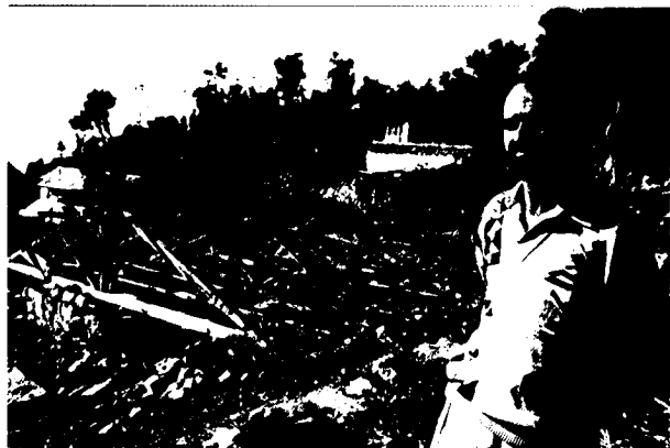
FIGURE 1: Kashmiri health care provider in front of collapsed Health Facility. This was the typical scene of destruction for many hospitals and health care facilities after the October 8 earthquake.
