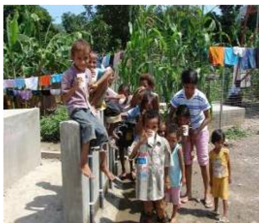
Children having access to safe drinking water
