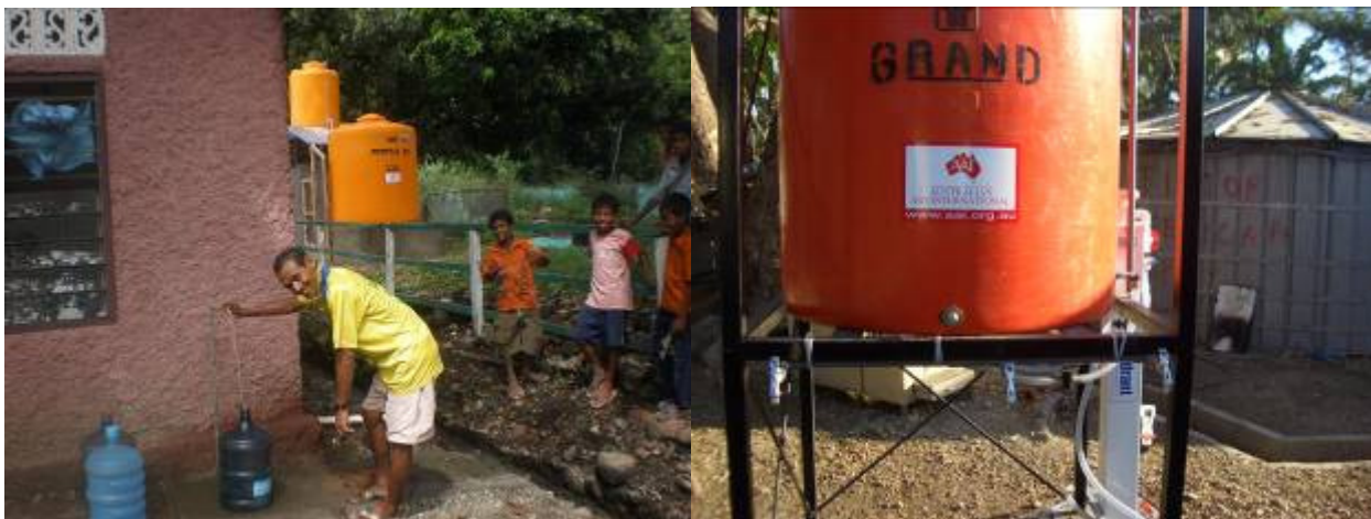
Safe water purification projects in remote communities in Timor-Leste
